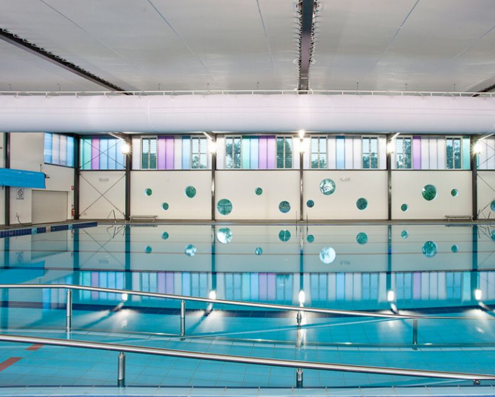
Pictured: Dalby Aquatic Centre | Project completed while at Liquid Blu
